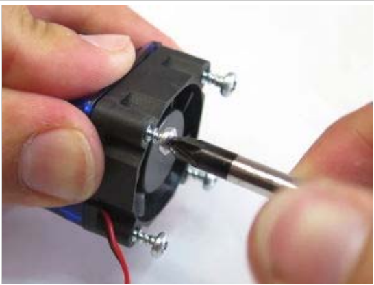
Screwing fan to duct.
